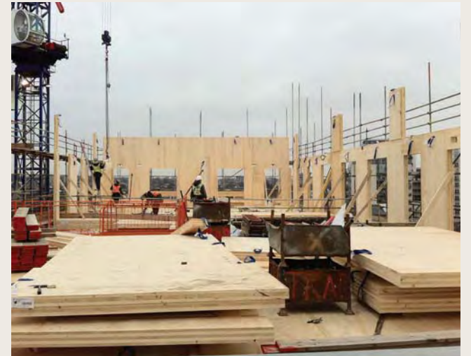
Panels with preformed windows are installed on the top floor.
